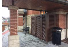
fully enclosed, planning for any future development of the property.3. Security and safety. Ground mounted mechancial equipment screening should be designed to provide total security, preventing the public from accessing the equipment accidentally
