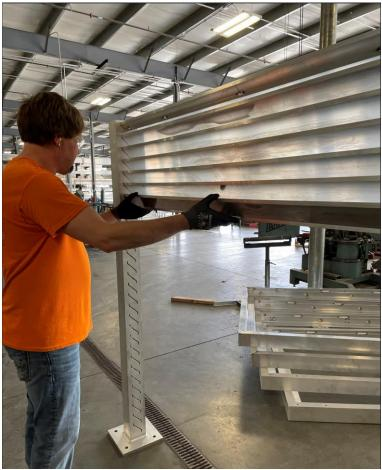
11. Once the louvers are installed you must install the vertical backstrap in between each bay. The louvers are all pre-drilled and the backstrap is pre-drilled. Start with the backstrap aligned with the top louver and install first rivet. The backstraps are labeled "top".
